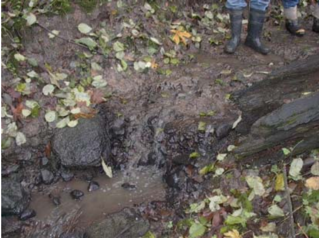
Photo: Erosion exposes boulders in stream bank in lower state park.
